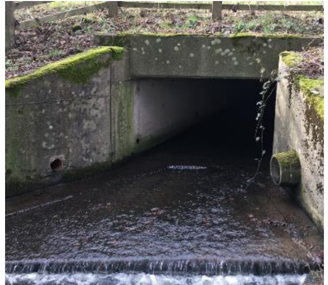
Figure 3-29 Shipperton Burn A1 Culvert (Outlet)
