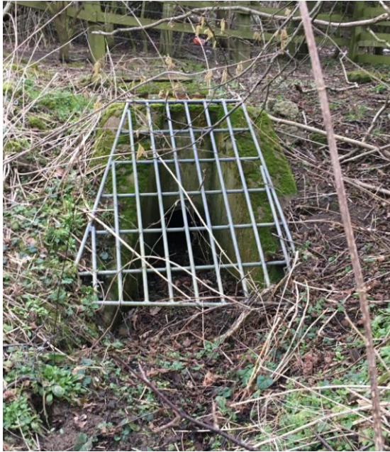
Figure 3-8 Denwick Burn A1 Culvert 2 Inlet
