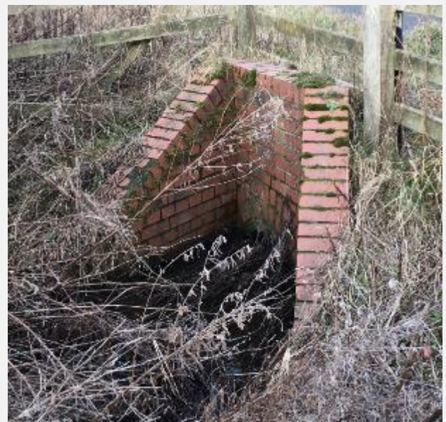
Figure 3-22 B6347 Eastern Culvert (Inlet)
