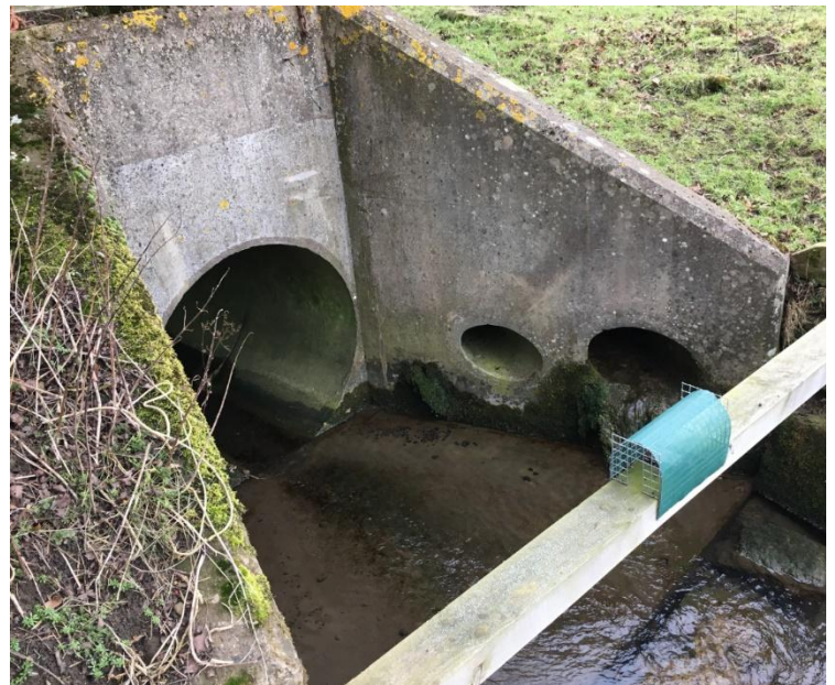
Figure 3-4 Denwick Burn A1 Culvert 4 Outlet
