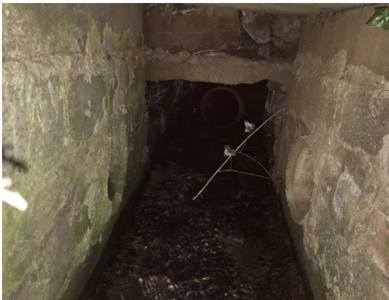
Figure 3-16 Farm Access Track Culvert along Tributary of White House Burn (Outlet)
