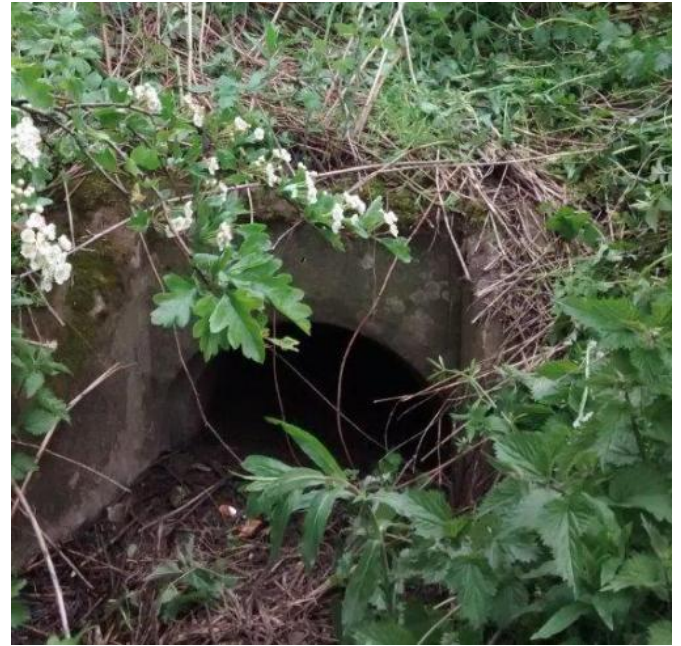
Figure 3-20 Southern Tributary A1 Culvert (Inlet)
