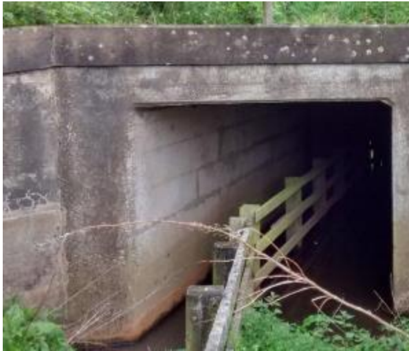
Figure 3-23 Western Tributary of Kittycarter Burn Culvert Underneath A1 (Inlet)
