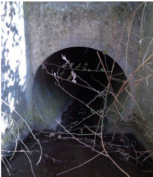
Figure 3-3 Denwick Burn A1 Culvert 4 Inlet
