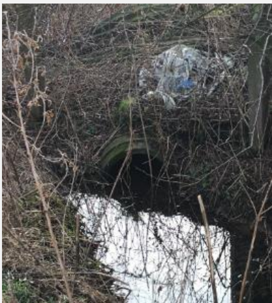
Figure 3-21 Small Access Track Culvert (Outlet)
