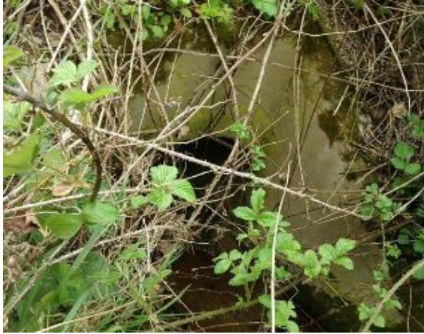
Figure 3-11 Denwick Burn A1 Culvert 1 Inlet
