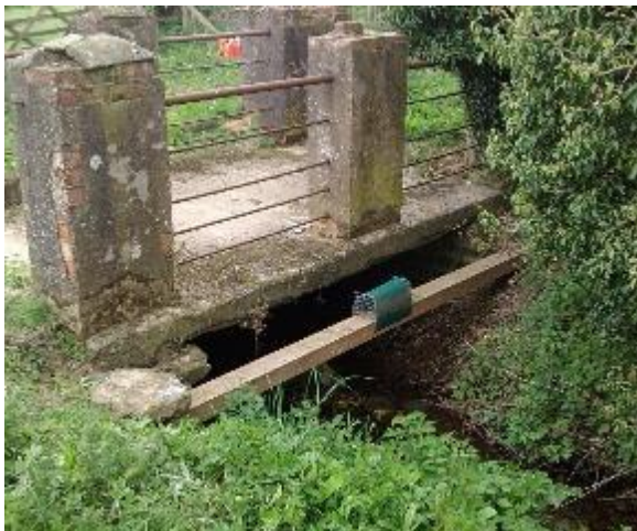
Figure 3-9 Farm Access Culvert 2 Inlet
