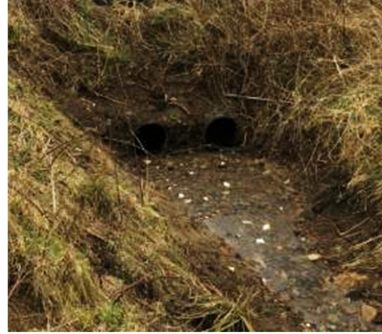
Figure 3-12 Farm Access Culvert 1 Inlet
