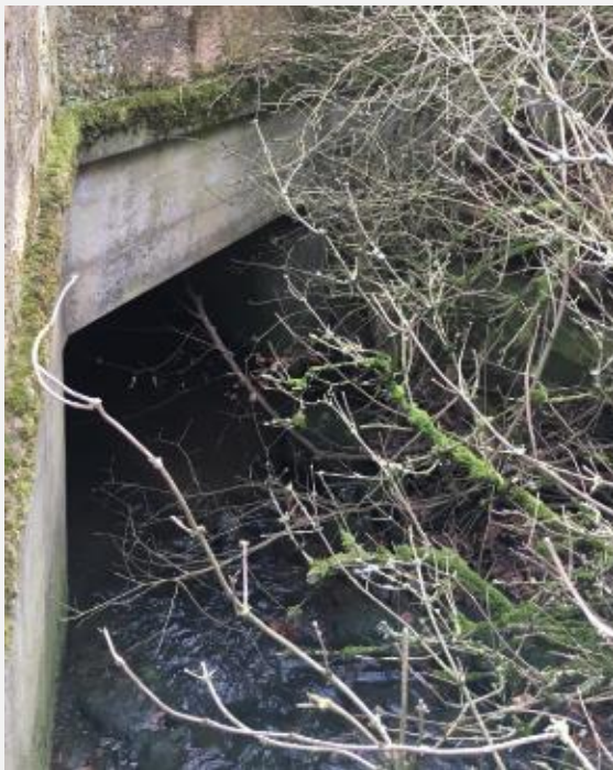
Figure 3-30 Shipperton Bridge (Inlet)
