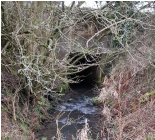
Figure 3-17 Culvert Underneath the B6341 (Inlet)
