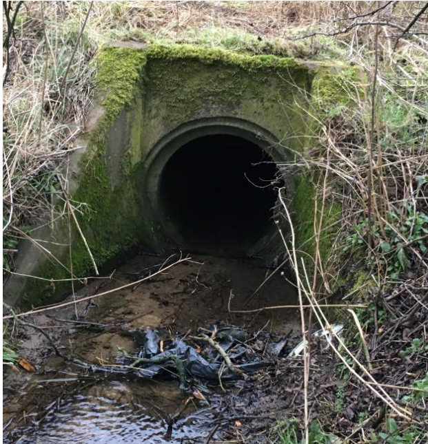
Figure 3-7 Denwick Burn A1 culvert 3 Inlet
