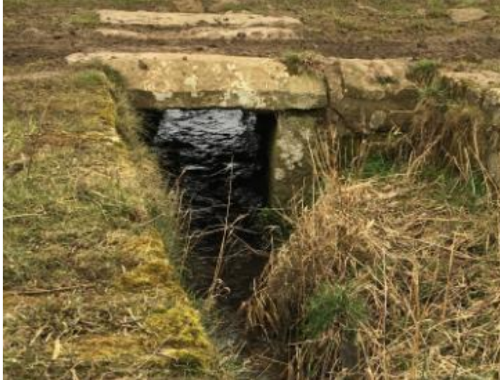
Figure 3-5 Public Right of Way Denwick Burn Crossing
