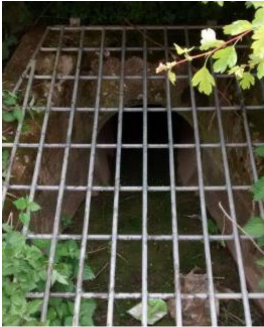
Figure 3-19 B6347 Western Culvert (Inlet)
