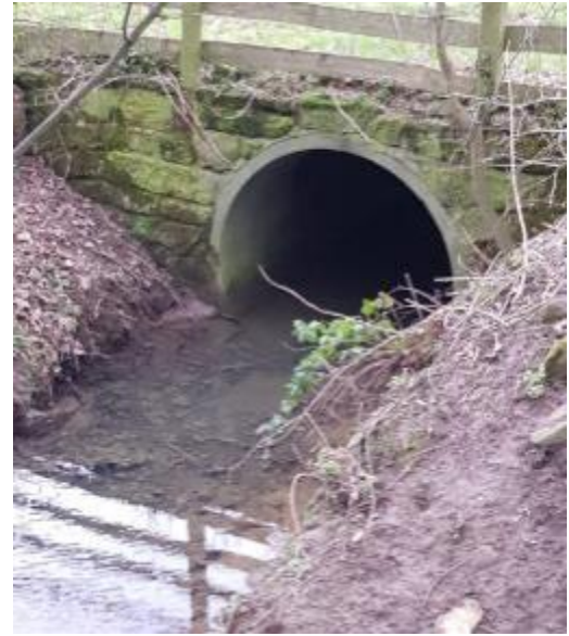
Figure 3-15 White House Burn Field Access Culvert (Outlet)
